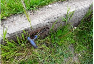
Finding: There is some evidence of rot in the timber sleeper Action: Monitor for any further deterioration and replace as required
