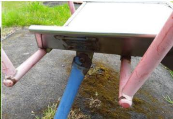
worn exposing the metal underneath which is rusting
