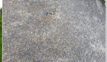
Finding: The safety surface under or around this unit has been damaged
