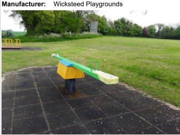
Finding: Parts of the steel on this item have corroded excessively and the metal has perforated in places
