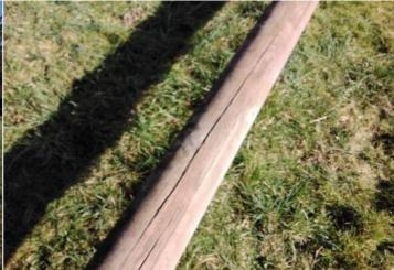
**Finding:** The timber has a number of splits/shakes or air **Action:** Monitor to ensure the splits do not cross through cracks and this may affect the stability or allow water ingress fixing points of the structure and/or cause any instability which will accelerate the rotting process
