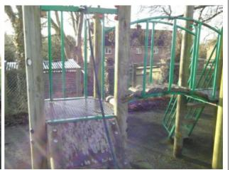
The unit is easily accessible and should have the appropriate barriers installed as the height of the unit exceeds 600mm Finding:
