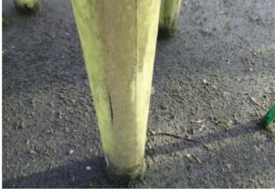
Finding: The timber has a number of air cracks apparent, the splits will have penetrated the preservative applied to the timber and allow
