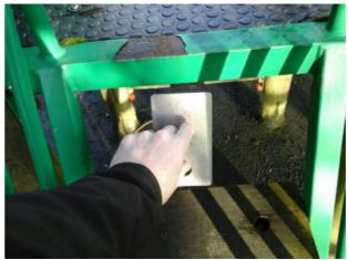
The item fails to meet the requirements of BS Action: EN 1176:2008 Part 1 4.2.7.2 head and neck entrapment in the barriers and/or steps Finding:
