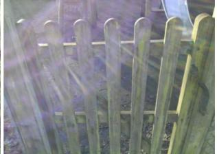
**Finding:** The opening between the gate and the post is **Action:** less than 12mm and could trap users fingers
