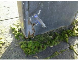
Finding: Parts of the steel on this item have corroded excessively and the metal has perforated in
