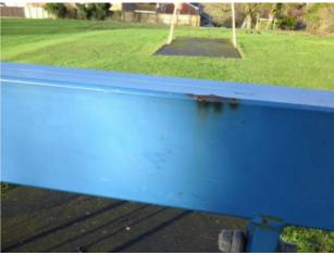
Finding: The paintwork on this item has been damaged or worn exposing the metal underneath which is rusting
