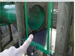
There are areas or parts of the timber on the **Action:** tunnel that have rotted Finding:
