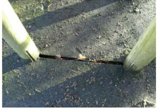
There are gaps opening between the surfacing and the edging surround or between the joints in the surfacing Finding:
