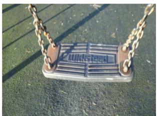
**Finding:** The swing seat connectors are loose **Action:** Tighten to secure
