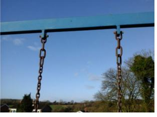
**Finding:** The bushes are showing signs of wear Action: Monitor for any further deterioration and replace as required
