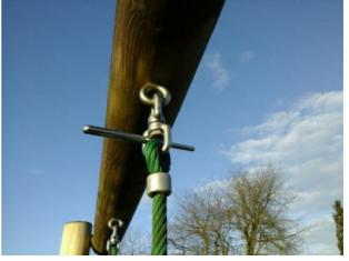
Finding: The connecting links are in excess of 8.6mm and less than 12mm and fail the requirements
