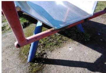
**Finding:** The paintwork on this item has been damaged or worn exposing the metal underneath which is rusting
