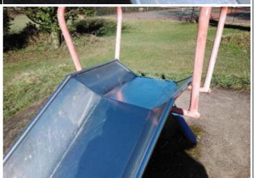
**Finding:** The slide start section incline is not in the direction **Action:** Monitor - No remedial work recommended of travel; it should slope towards the direction of the sliding surface to meet the requirements of BS EN 1176 Part 3
