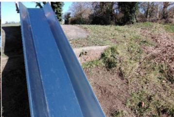
Finding: The timber sleeper forms a hard object within the Action: Monitor - No remedial work recommended impact area of the equipment in contravention of the requirements of BS EN 1176 Part 1
