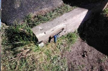
Finding: There is some evidence of rot in the timber sleeper Action: Monitor for any further deterioration and replace as required
