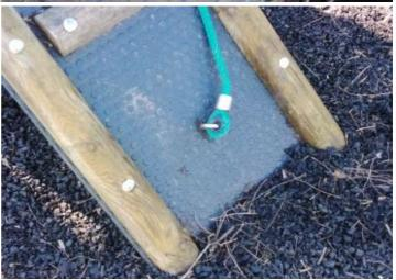
Finding: The ropes/nets are worn/damaged in places
