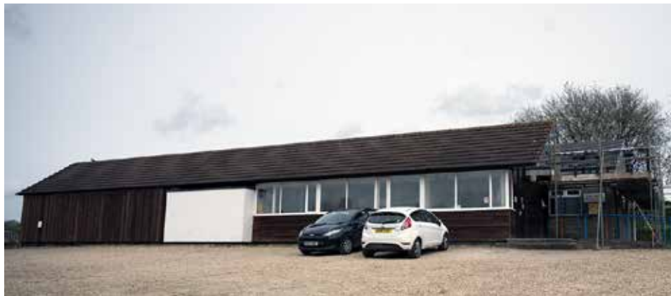
West Meon Village Hall with scaffolding. Photo: A Annabel
